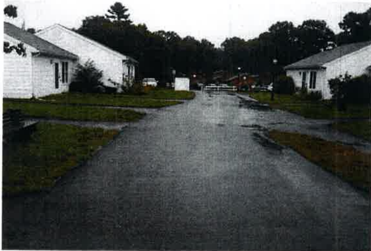
The central roadway running between the two rows of buildings was full fully resurfaced in 2013 as well.
