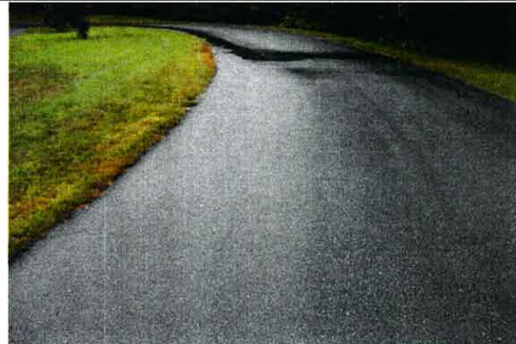
The loop roadway was fully resurfaced in 2013 and remains in generally good observable condition.
