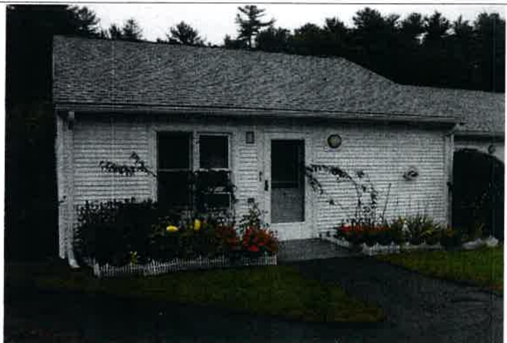
View of typical building/unit front elevation with original (1995) vinyl siding; Harvey vinyl-framed, double-hung windows; half-lite metal-clad entry doors; and recently (2016) installed architectural (dimensional) asphalt shingle roof;
