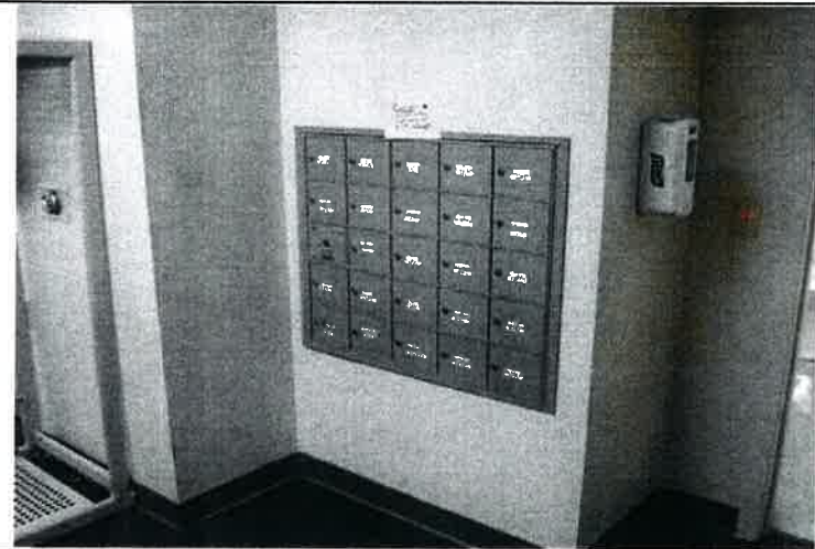
The community building hallway also features a recessed-aluminum cluster mailbox panel that was newly installed in 2014.
