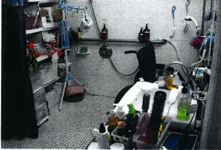
The 14-F bathroom also features a fully tiled roll-in shower stall with compliant center-mounted valve control and shower hose with hand-held shower head; however this sink is also positioned too low.
