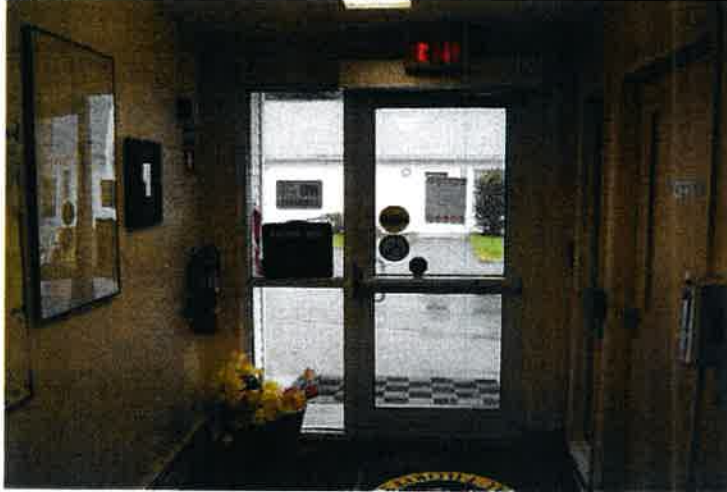
The community building features painted drywall walls and ceilings, recently (2018) installed carpet-tile flooring; and power assist door openers and the front and rear entrance doors.
