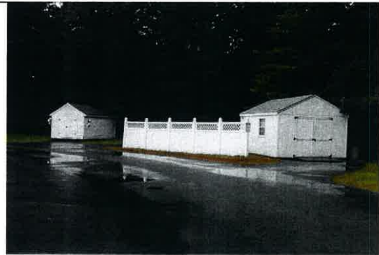
View of the two wood-framed maintenance sheds and vinyl privacy-screen fencing that hides additional maintenance equipment. The near shed was recently installed in 2015. The far shed dates to the 1995 construction.
