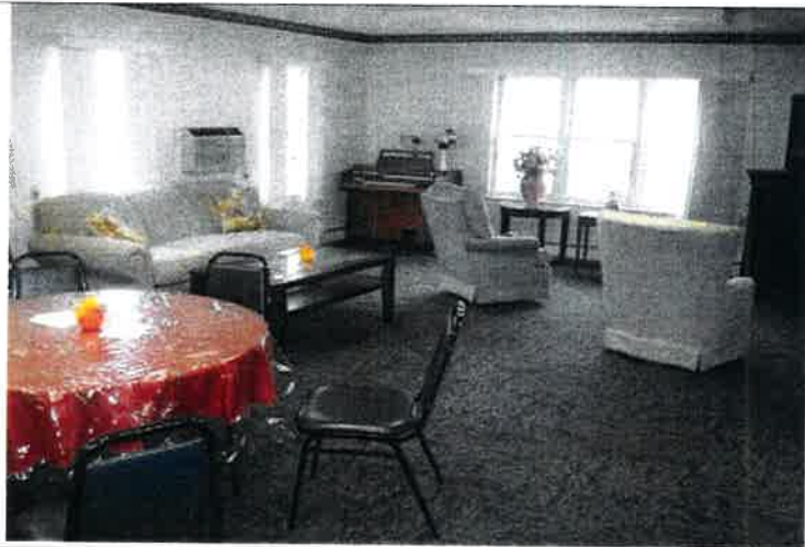
View of the community room finishes and furnishings with new (2018) carpet tile flooring; upholstered couches and lounge chairs; activity/dining table; and stackable padded chairs that were all newly installed in 2014.
