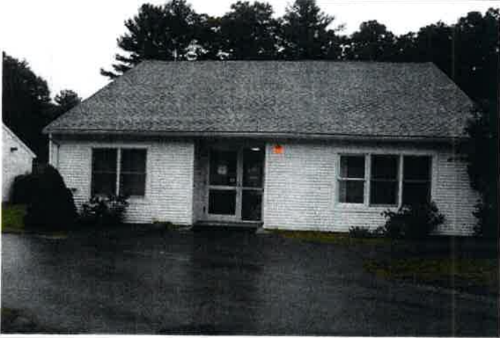
View of the community building front elevation with commercial storefront-style, aluminum and glass entry door and adjacent fixed glazing panel.
