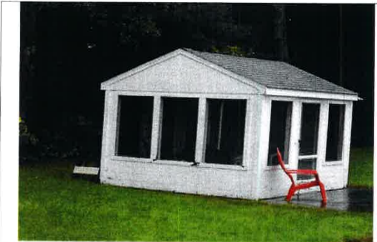
The ageing "Screen House" enclosed patio structure dates to the original 1995 construction as well and exhibits visible age and weather related siding, trim, door, and frame rot.
