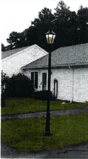
The walkways are lit by a series of post lanterns that were all upgraded with new energy-efficient LED fixtures in 2016.
