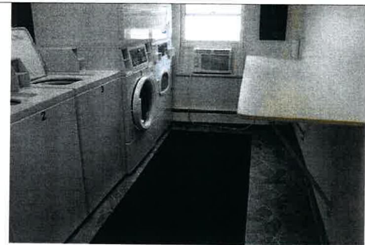
The wall-mounted clothes folding table was installed at the request of the residents; however it restricts compliant access to, and maneuvering room around, the accessible floor-mounted, front-loading washer dryer pair.
