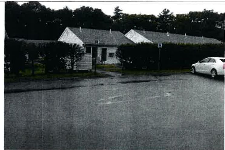
View of typical accessible parking stalls with compliant standing signs; however the striping, access aisle and surface symbols have faded considerably and are in need of near-term re-striping.
