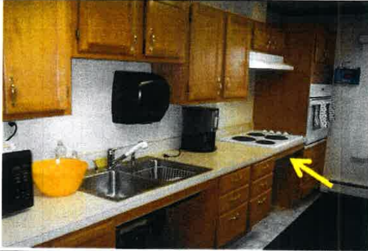
The community room kitchen also features; a forward-facing, roll-under cooktop, rangehood, and wall-oven; however there is no compliant apron-mounted rangehood control switch.
