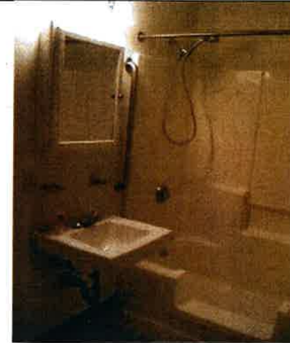
Standard unit bathrooms feature painted drywall walls and ceilings; vinyl-sheet flooring; wall-mounted porcelain sinks and wood medicine cabinets; low-flow toilets; and fiberglass tub-shower assemblies with sidewall cutouts.
