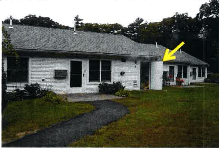
View of typical building/unit rear elevation with similar siding, roof, windows, and concrete patios. Each building also features a central mechanical room accessed through a flush-metal service door (arrow).
